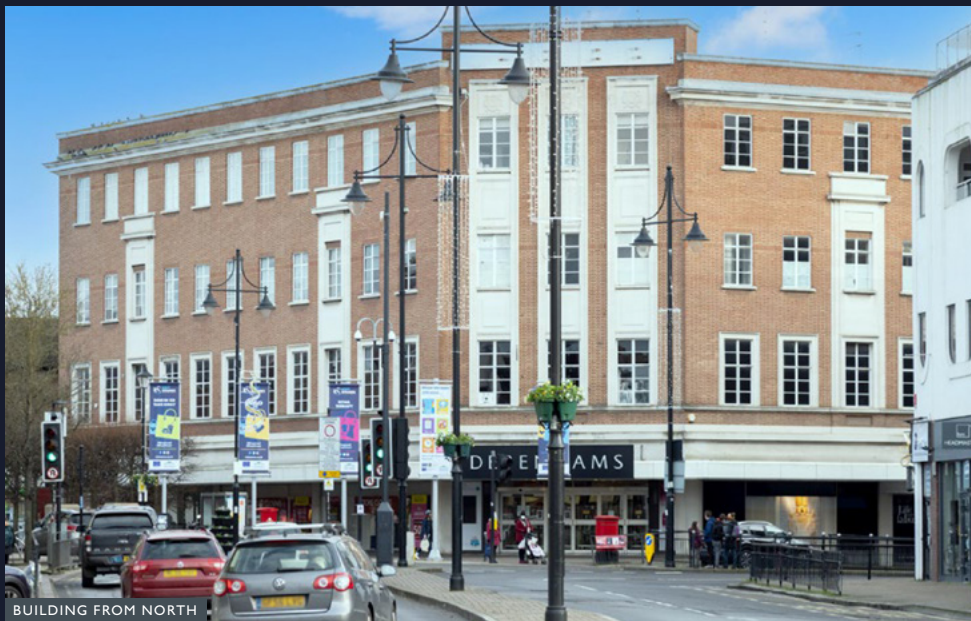
BUILDING FROM NORTH
