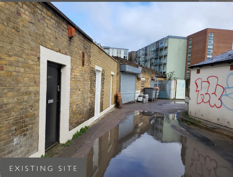
EXISTING SITE - VIEW FROM RYE LANE
